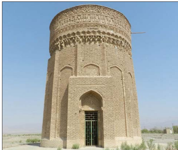
The Southern Façade of Mehmandūst Tower
